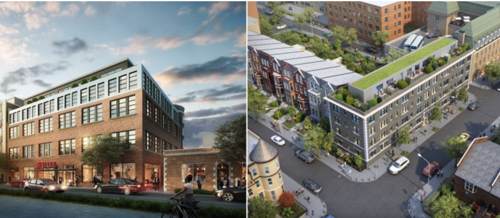
PHOTO: EucKal Apartments, Jubilee Housing
